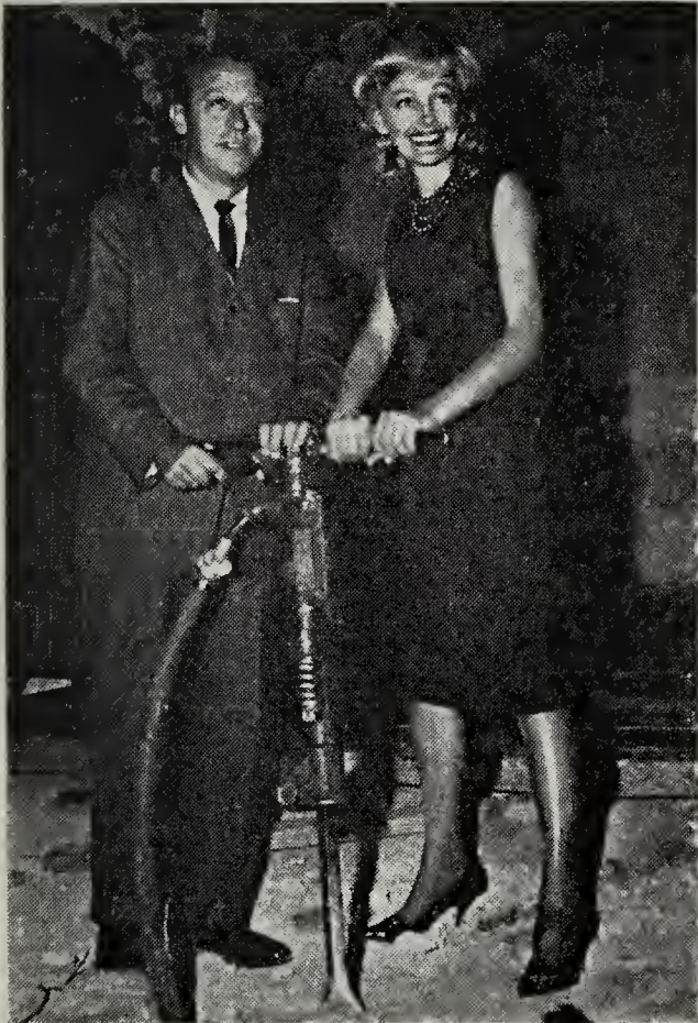
Pat Notaro, western zone manager for Stanley Warner Theatres, shows actress Virginia Grey how to use a jack-hammer during the $250,000 remodeling of the New Warner Hollywood, which will become Hollywood's newest first run house after nine years as the home of Cinarama. Miss Grey co-stars in U-I's "Back Street," which will reopen the theatre with a premiere on Oct. 26.
